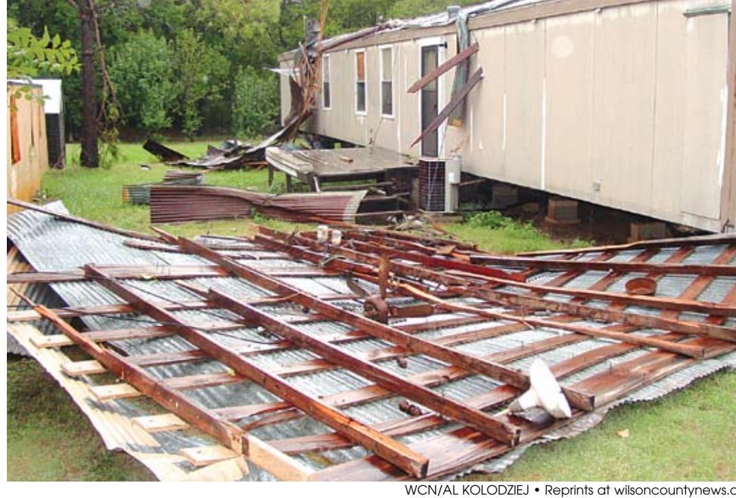
A home off Bernhardt Road near Calaveras Lake is impaled with several pieces of lumber, while the roof of a storage building lies in the yard. High winds and heavy rain resulting from the remnants of Hurricane Dolly moved through the area on the morning of July 24, causing tornado warnings to be issued.
